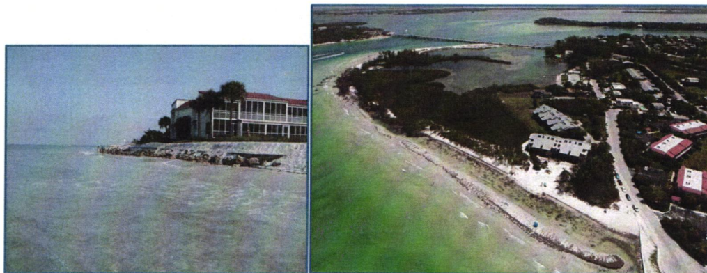
Erosion Near Longboat Pass
