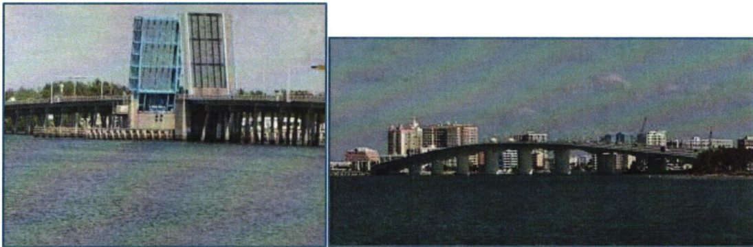
Cortez Bridge (Left); John Ringling Bridge (Right)
