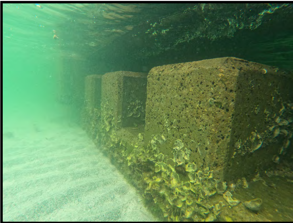
Photograph 12. Groin Structure (South Side)
