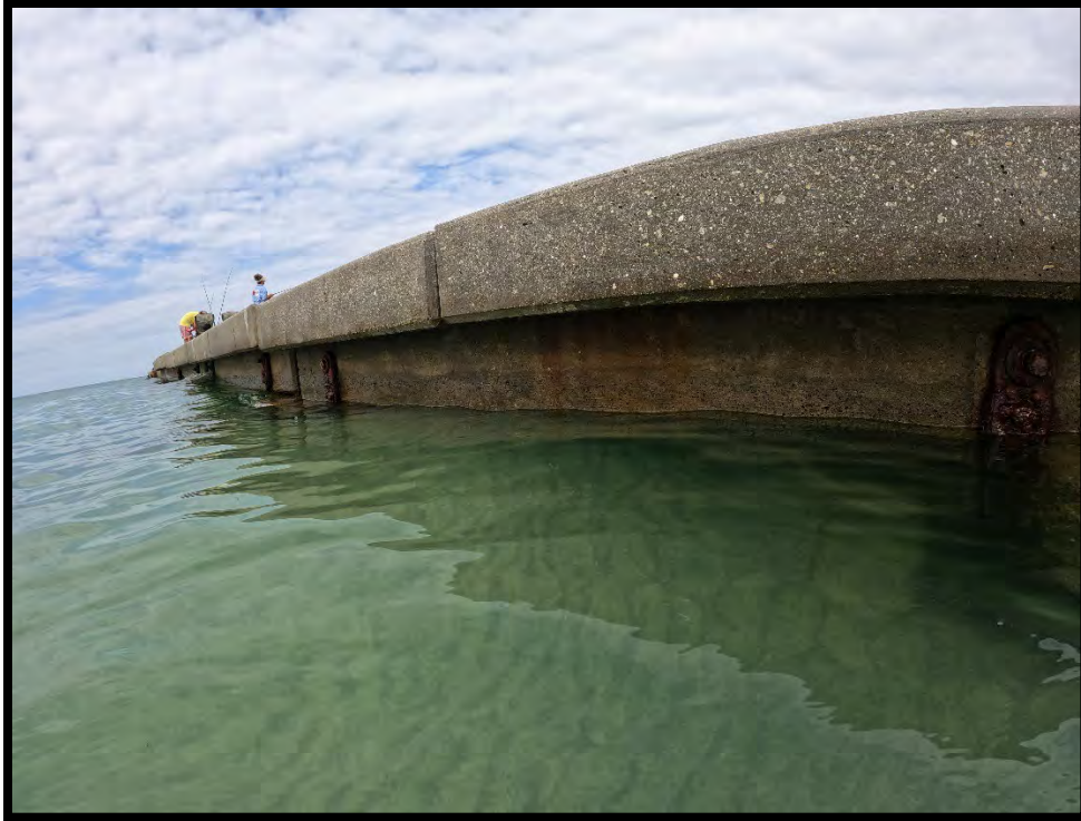
Photograph 11. South Side of Groin Facing West
