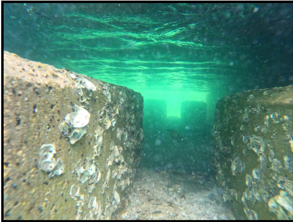
Photograph 13. Facing North Underneath Groin Structure
