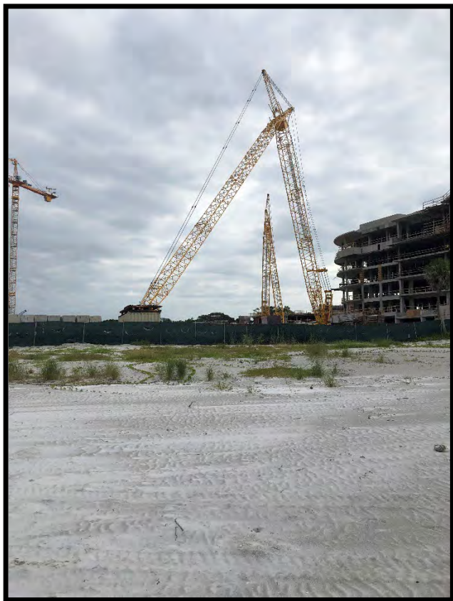
Photograph 6. Facing Dunes and Hotel Construction to the East
