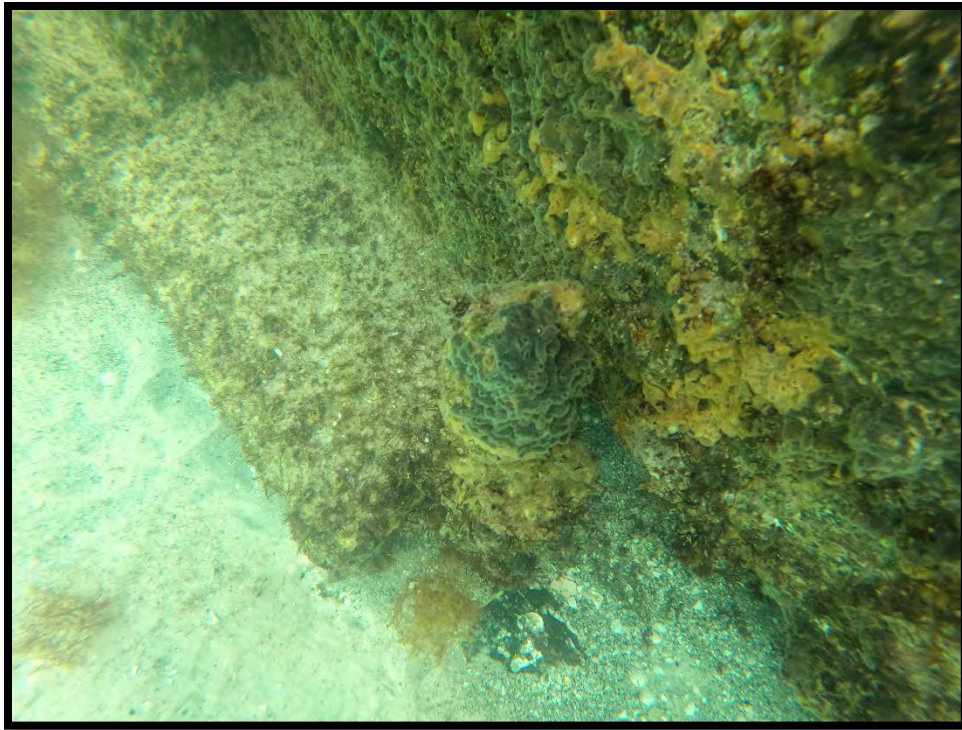
Photograph 15. Yellow and Blue Encrusting Sponges on Groin Structure
