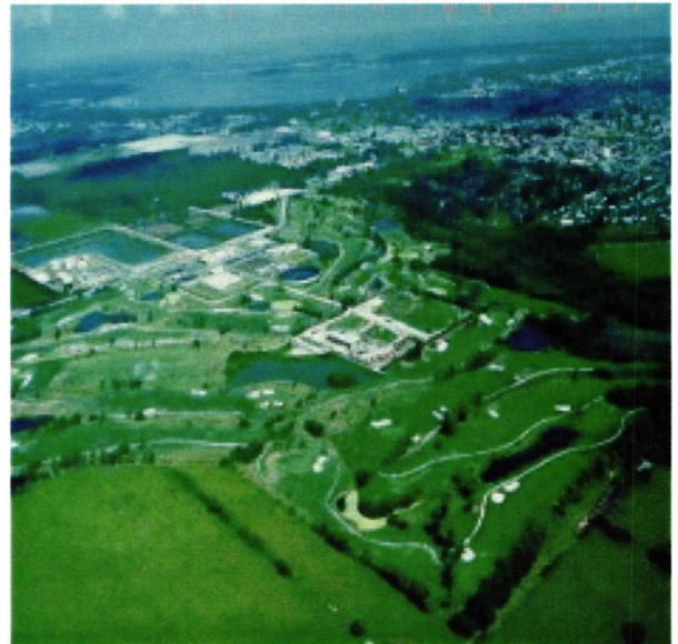
Manatee County Southwest Regional Treatment Plant
