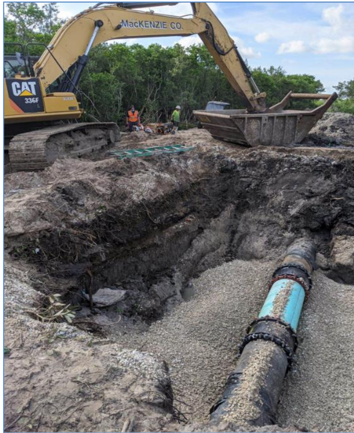
Figure 1-1 Repair of Existing Force Main Within Mangroves
