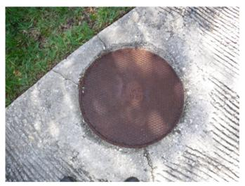
Cracks adjacent to manholes may contribute to infiltration of saltwater into utility conveyance systems in areas of regular tidal flooding.
