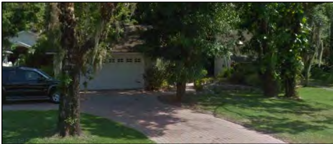
Figure 2: Slab on Grade Structure on Phillippi Creek Bank
