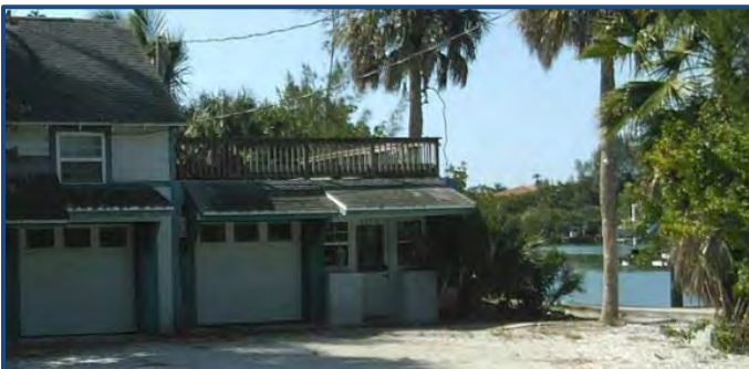
Figure 2: Slab on Grade Structure Adjacent to Waterway
