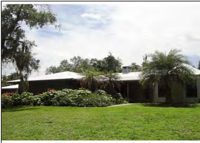
Figure 2: Slab on Grade, Concrete Block Structure
