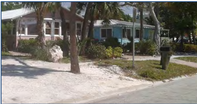
Figure 2: Minimally Elevated Structure Adjacent to Coastal Beaches
