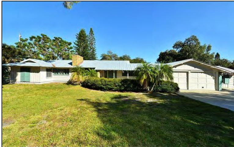
Figure 4: Wood Frame Structure
