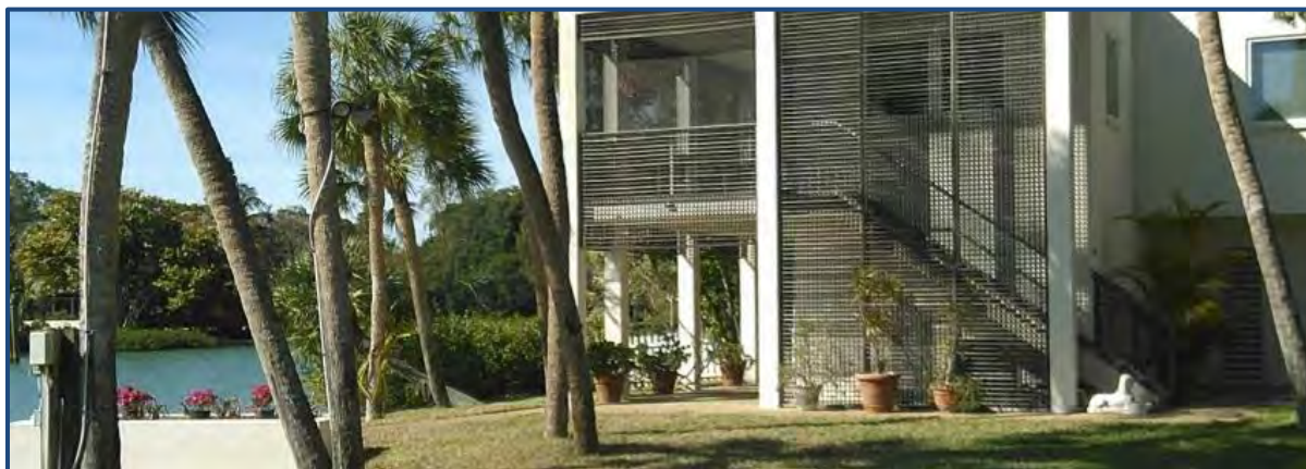
Figure 4: Structure Adjacent to Waterway
