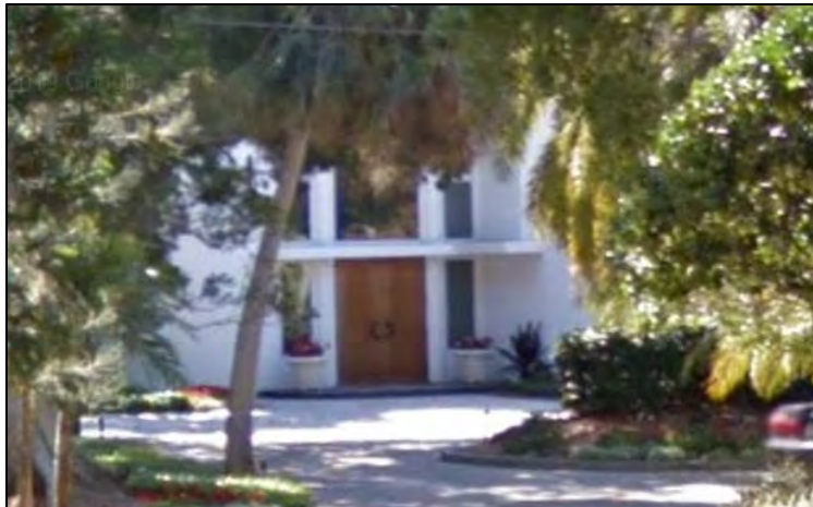
Figure 4: Slab on Grade Structures (Google Maps)
