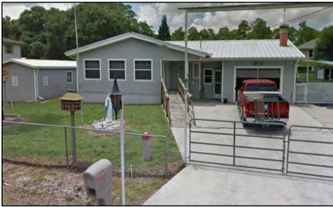
Figure 2: Elevated on Stem Wall Structure
