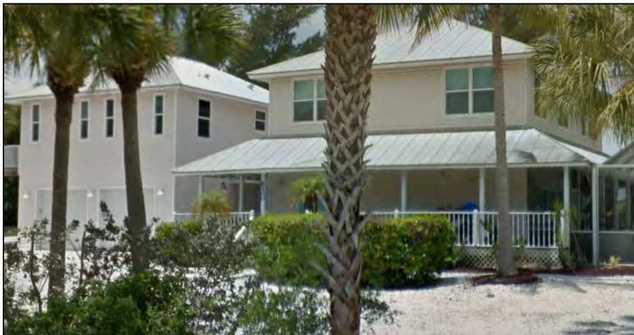
Figure 4: Average Elevated on Post Structure
