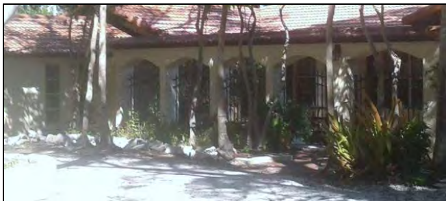
Figure 2: Masonry, Slab on Grade Structures
