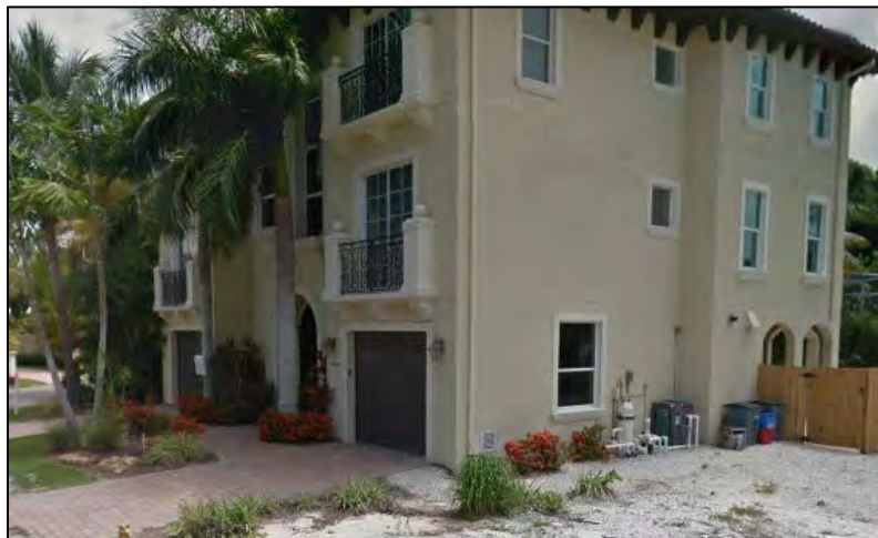
Figure 4: Example of Elevated on Post Structure
