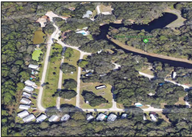
Figure 2: Overhead View of Structures (Google)
