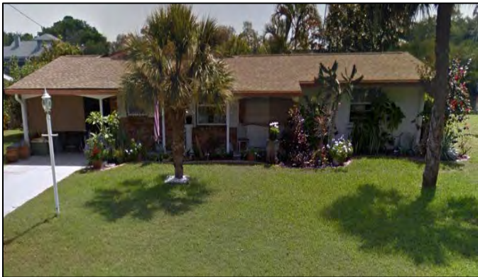
Figure 2: Slab on Grade Structure on Phillippi Creek Bank
