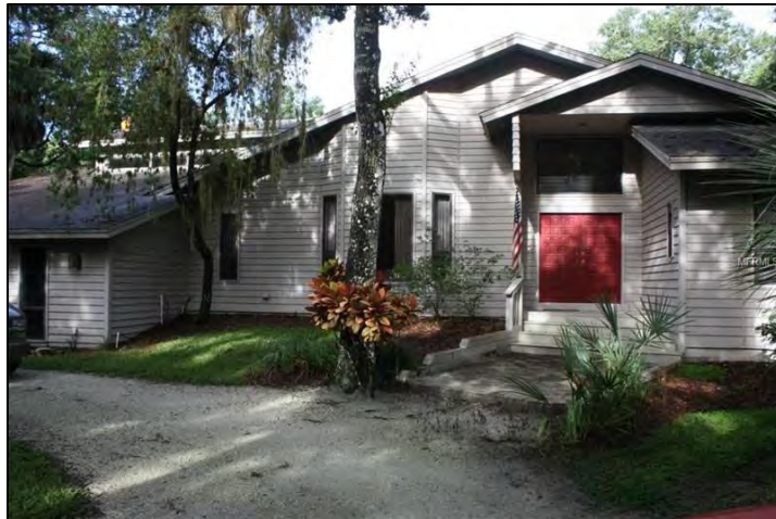
Figure 4: Elevated slab on stem wall with fill Raised Slab on Grade Structure
