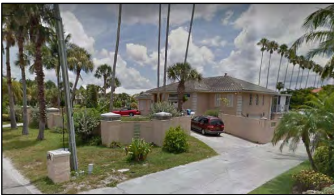
Figure 2: Structure Elevated on Stemwall Structure
