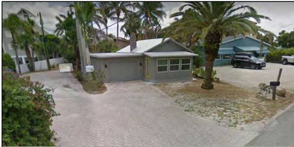
Figure 4: Slab on Grade Structures
