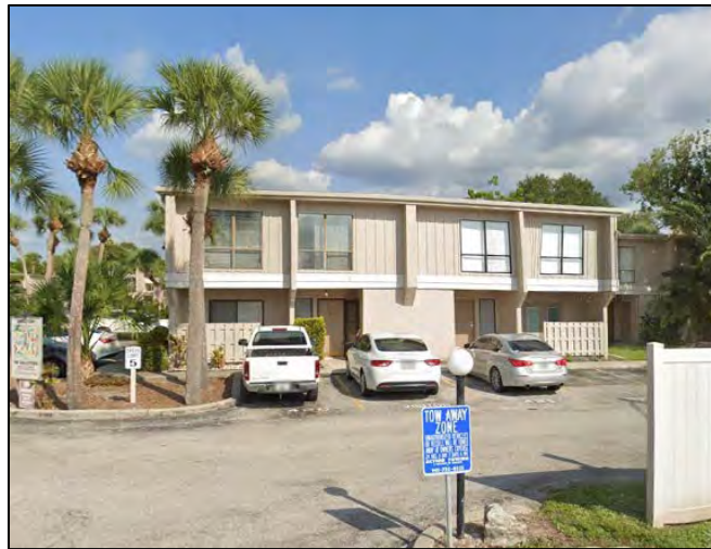
Figure 4: Slab on Grade Condominium Structures (from Google maps)
