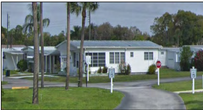
Figure 2: Mobile Home Structures
