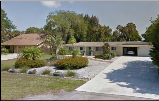
Figure 2: Slab on Grade Structures
