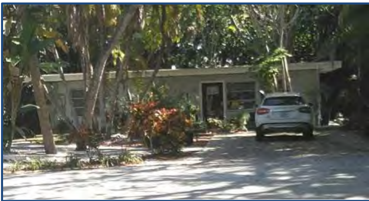
Figure 2: Slab on Grade Structures
