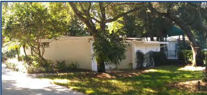
Figure 2: Slab on Grade Structures
