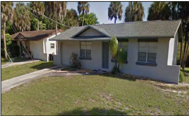
Figure 2: Concrete Masonry Structure
