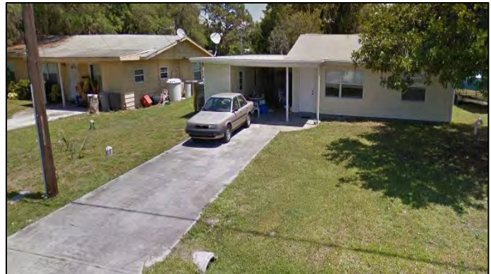
Figure 4: Slab on Grade Structures
