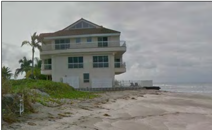
Figure 2: Elevated Coastal Structure
