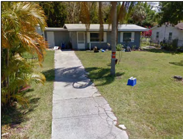
Figure 2: Slab on Grade Structures
