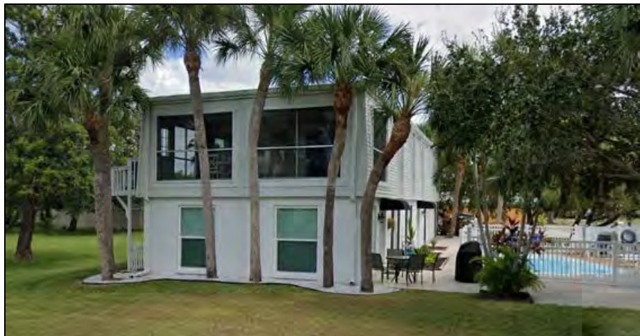
Figure 4: Slab on Grade Structure (Google Maps)
