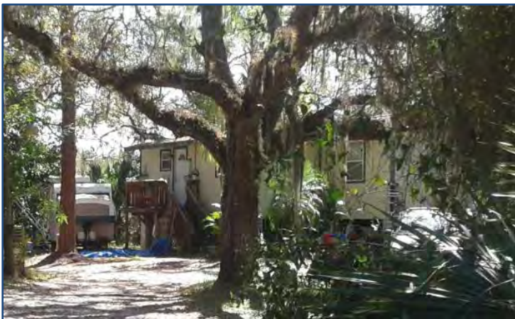
Figure 2: Wood Frame Structure
