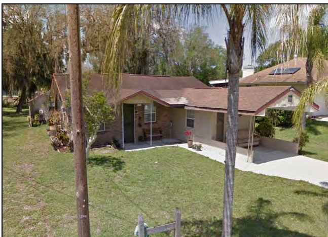
Figure 2: Concrete Block Structure
