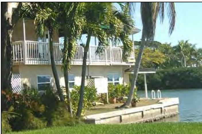
Figure 2: Slab on Grade Structure Adjacent to Waterway
