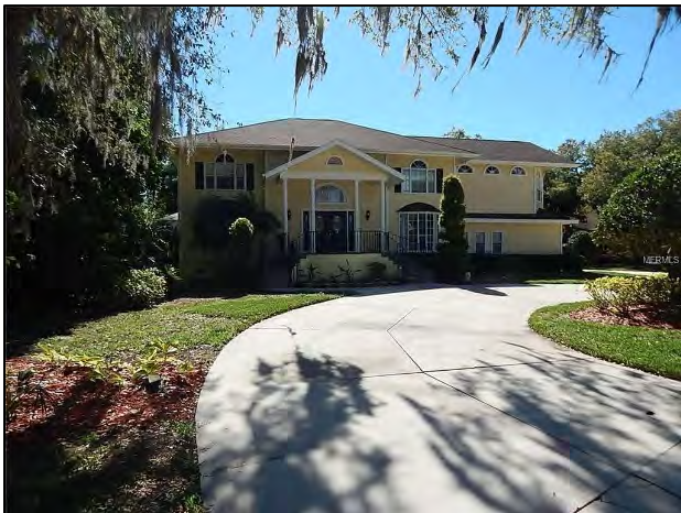
Figure 2: Wood Frame Structure
