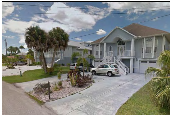
Figure 4: Average Elevated Foundation Wall with Enclosure Structure
