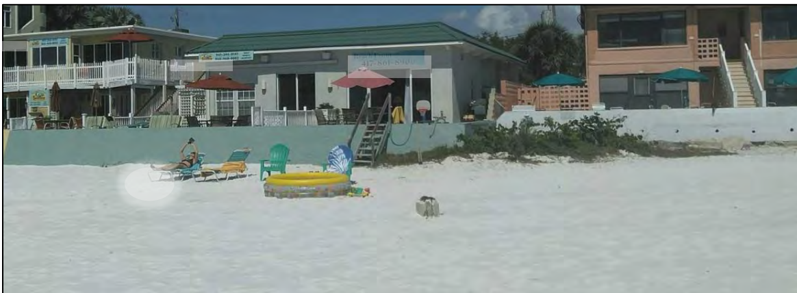
Figure 4: Minimally Elevated Structure Adjacent to Coastal Beaches
