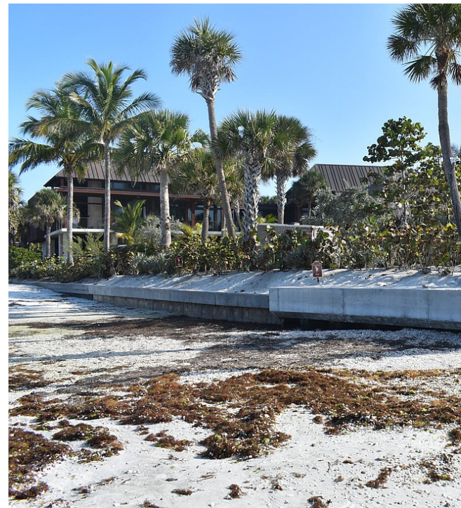
Seawalls at 6633 Gulf of Mexico Drive and 6541 Gulfside Road.
