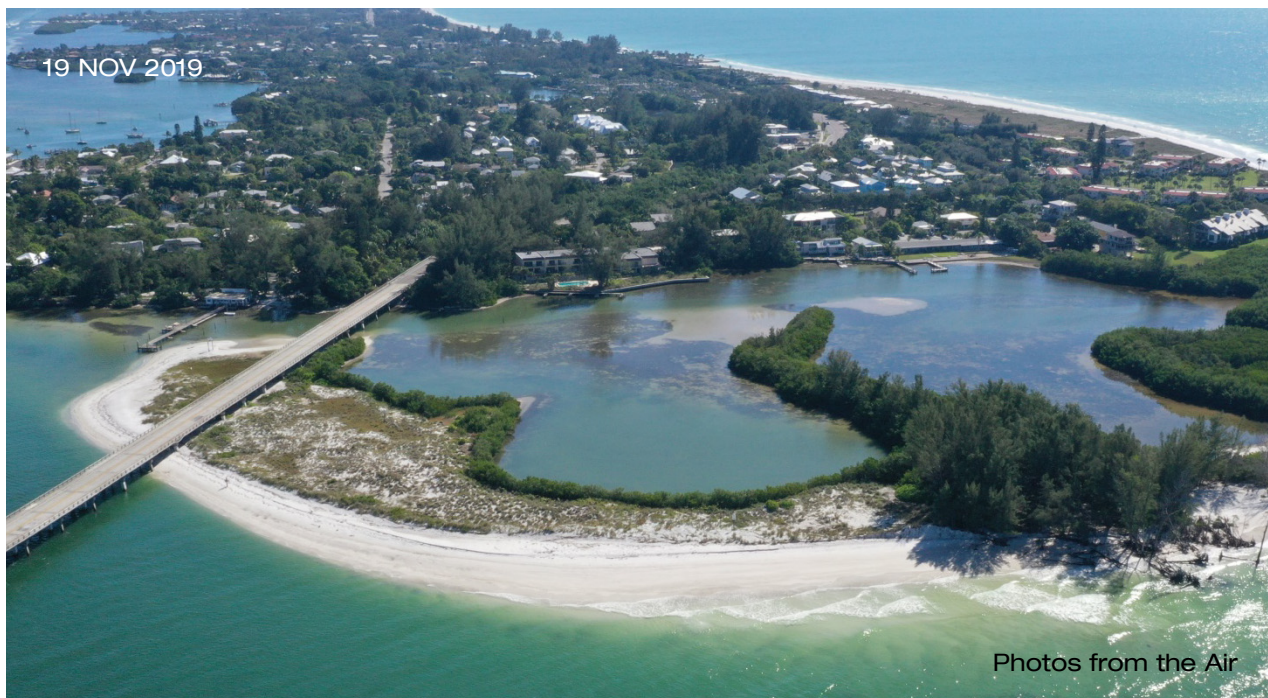
Figure 3.2 November 2019 condition of the Greer Island Longboat Pass shoreline.
