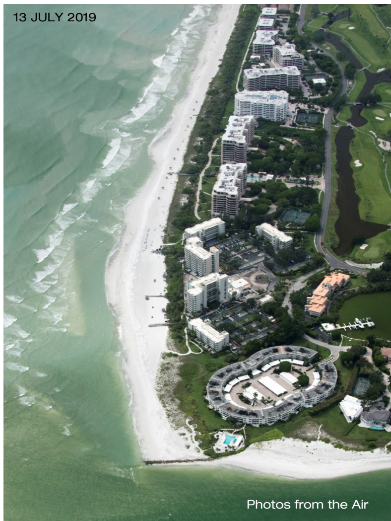
Figure 3.5 Condition of the Gulf shoreline from the Sanctuary Condominium (R-25) to New Pass (R-29) in Beach Segment #9 in Longboat Key, FL.
