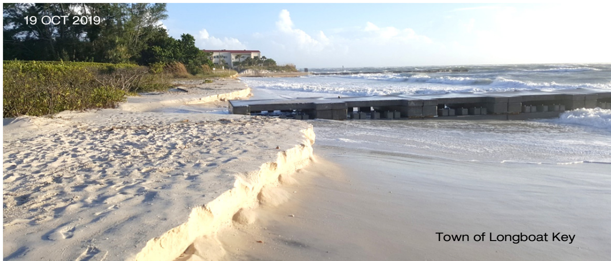
Figure 3.3 October 2019 eroded beach conditions in the vicinity of the North End Permeable Adjustable Groins (R-44 in Manatee County) on Longboat Key. The northern PAG is shown in the foreground.
