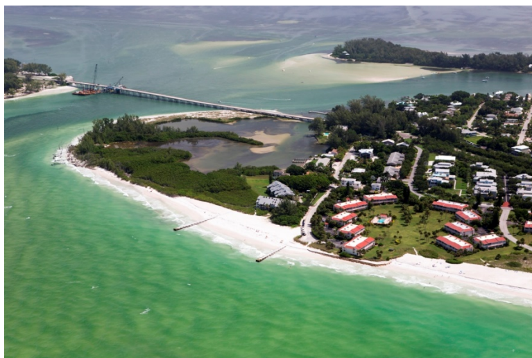
Figure EX-2 Aerial view of the North Shore Road Permeable Adjustable Groins (PAGs) shortly after completion, and the north end of Longboat Key at Greer Island and Longboat Pass. (6 Aug 2015, Photos from the Air).
