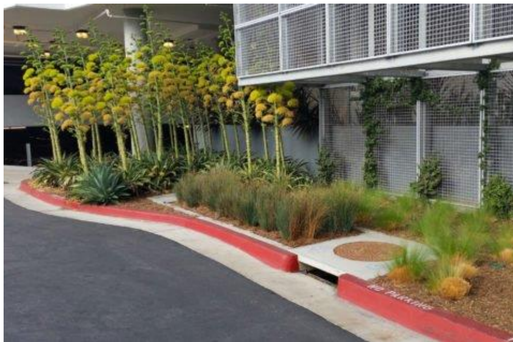
Figure 5: Installed Modular / Linear Wetland System
