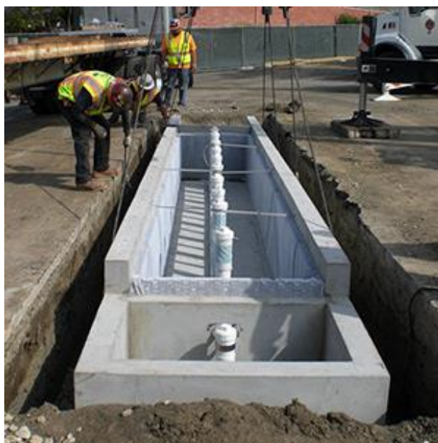
Figure 6: Installation of Modular / Linear Wetland System
