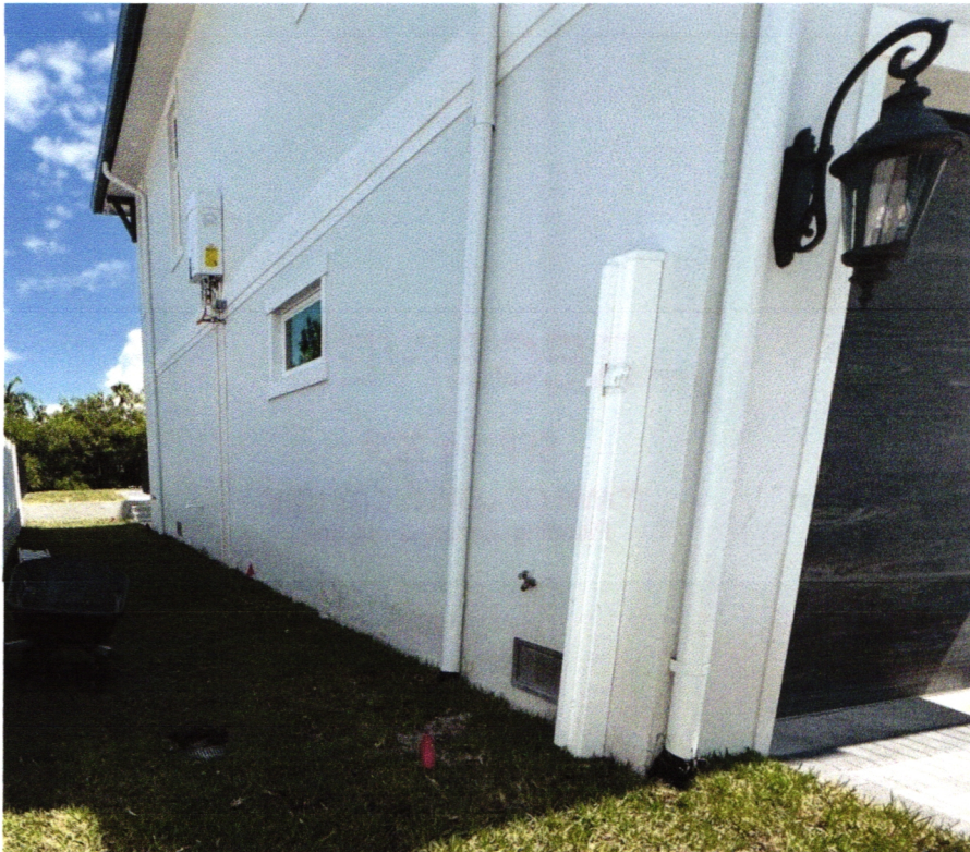
(08/27/2024) Left Side View, 2 Smart Vents, Elevated Tankless Water Heater=13.6'
