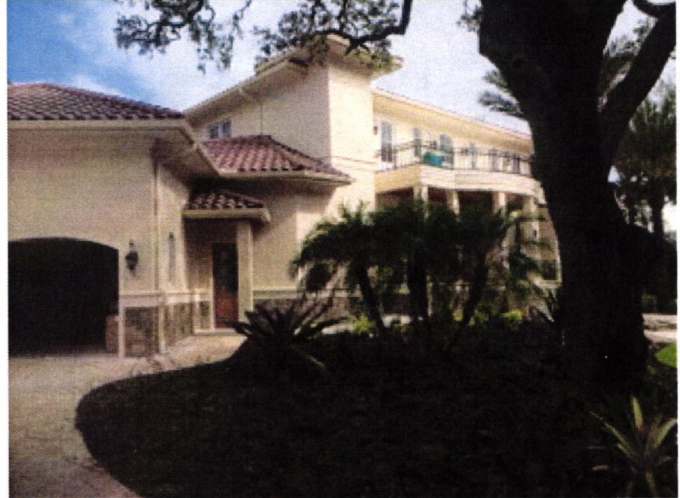
GARAGE LEFT SIDE VIEW WEST VIEW 11/20/2015
