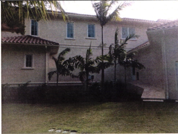
LEFT SIDE VIEW NORTHWEST VIEW 11/20/2015
