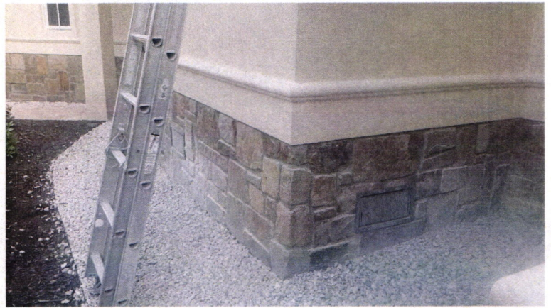
FOYER AND ELEVATOR SHAFT 1 SMART VENT MODEL 1540-520 IN EACH AREA 12/07/2015
