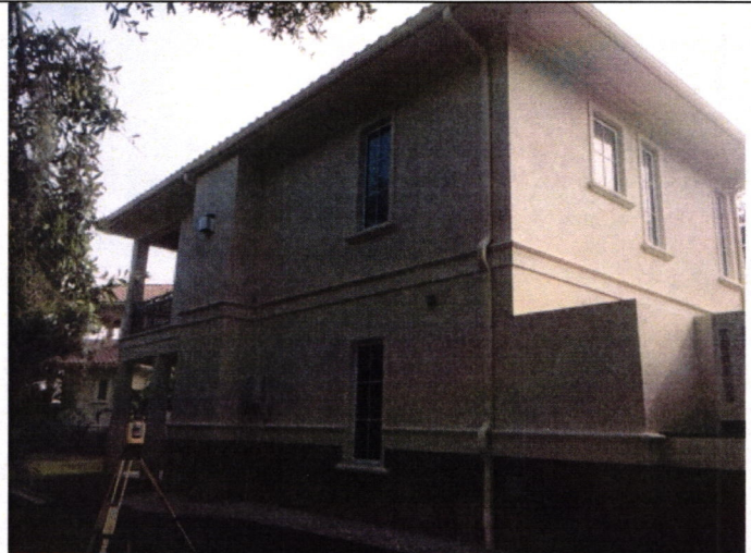
REAR AND LEFT VIEW NORTHWEST CORNER VIEW 11/20/2015
