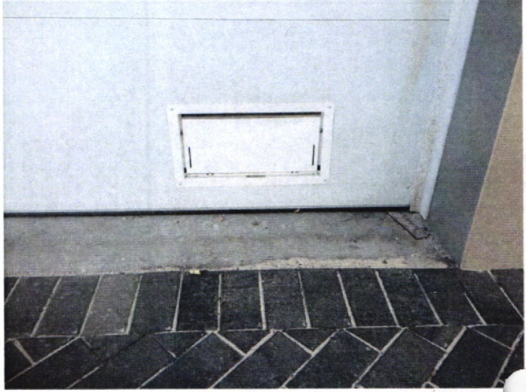
TYPICAL SMART VENT MODEL 1540-524 IN GARAGE DOOR
