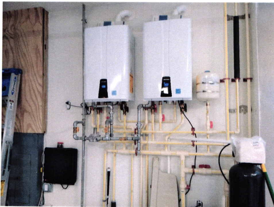
(06/13/2019) Tank Less Hot Water Heaters Located in Garage
