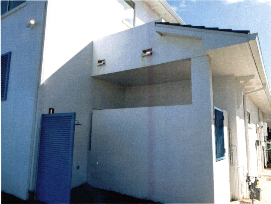
(11/14/2024) View of Elevated AC Platform=21.9' with Elevated Pool Equipment Enclosure Below on Left Side in Rear
