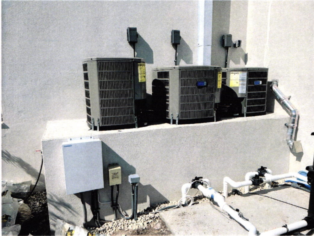
(03/29/2022) Elevated AC Units on Left Side of House
