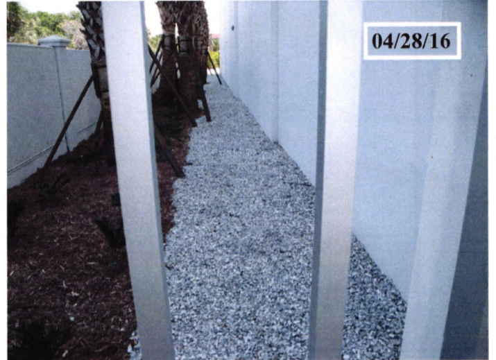
RIGHT SIDE VIEW LOOKING EAST
