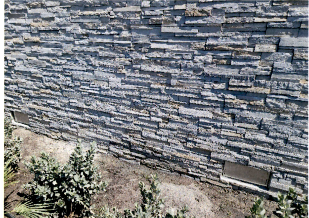
(03/03/2025) 3 Smart Vents in Garage Walls in Front
