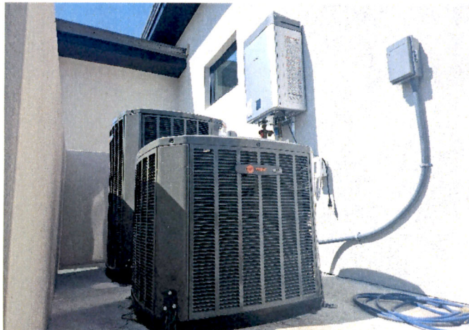
(03/03/2025) Elevated AC Platform=12.4'. Tankless Heater on Wall=16.3'
