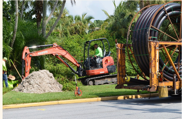
Photo of Wilco Electrical crews working in Longbeach Village (the Observer)
