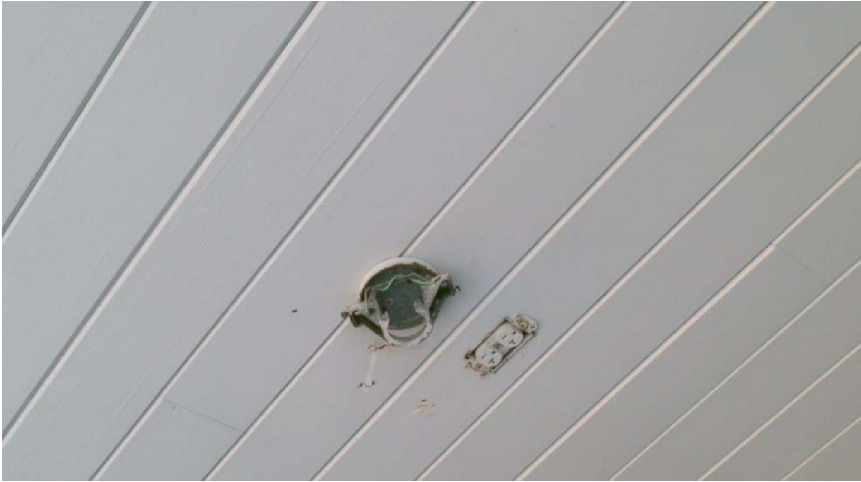
Exposed wiring at removed fixture
