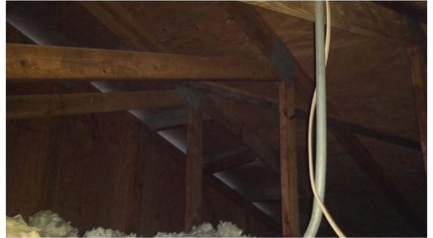
Inefficient insulation at ceiling. No insulation at roof deck
