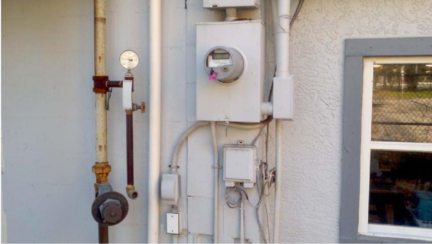
Valves and fire riser are exposed rusting
