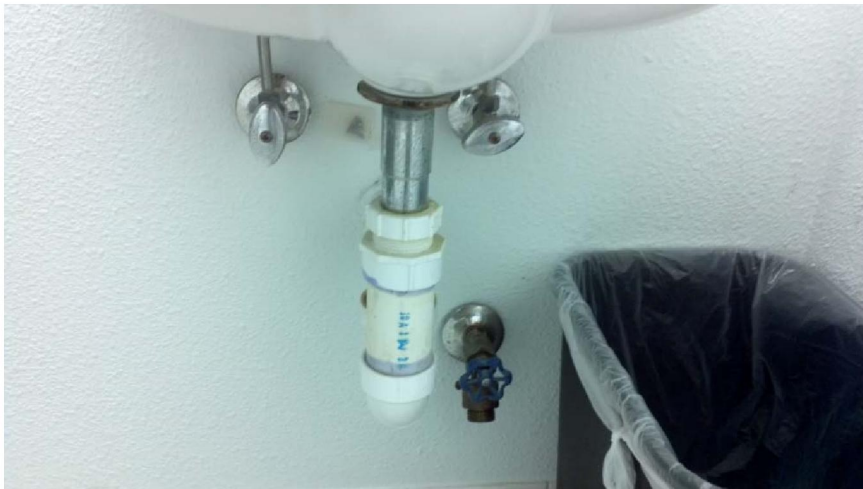
Piping is not protected per ADA
