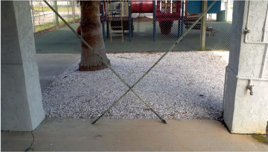
Lateral bracing is very loose and would be ineffective in a storm situation.
