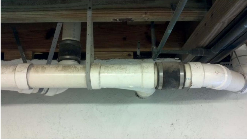
Extensive use of rubber couplings
