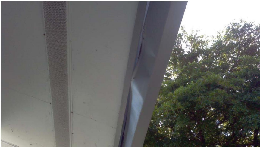
The Gutter is detached or bent at various locations
