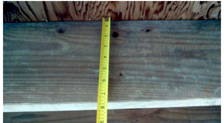
2x8 framing utilized for floor joist. 2x10 min is recommended for Assembly structures
