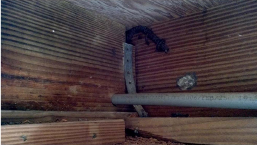
Requires proper hurricane straps and tie down
