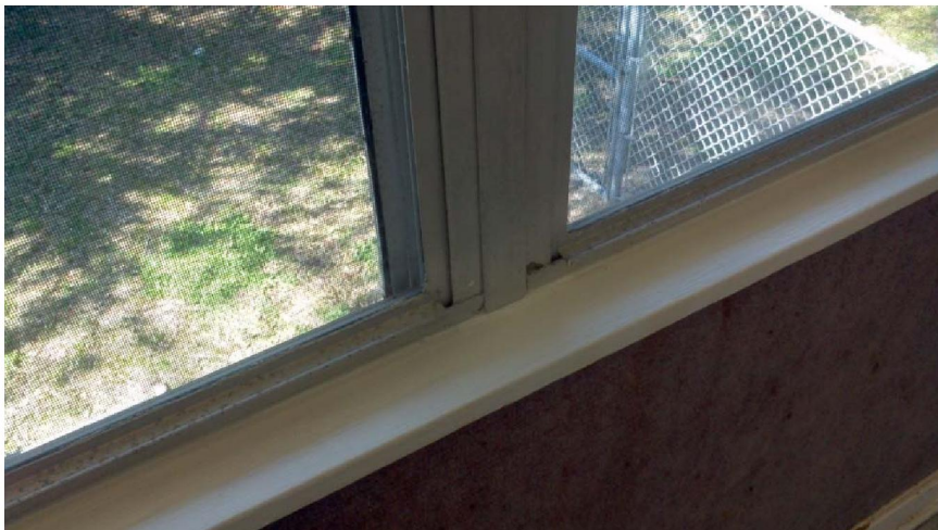
Windows/glazing does not meet current wind zone requirements
