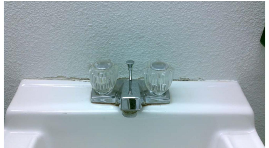
Fixtures should be lever controlled
