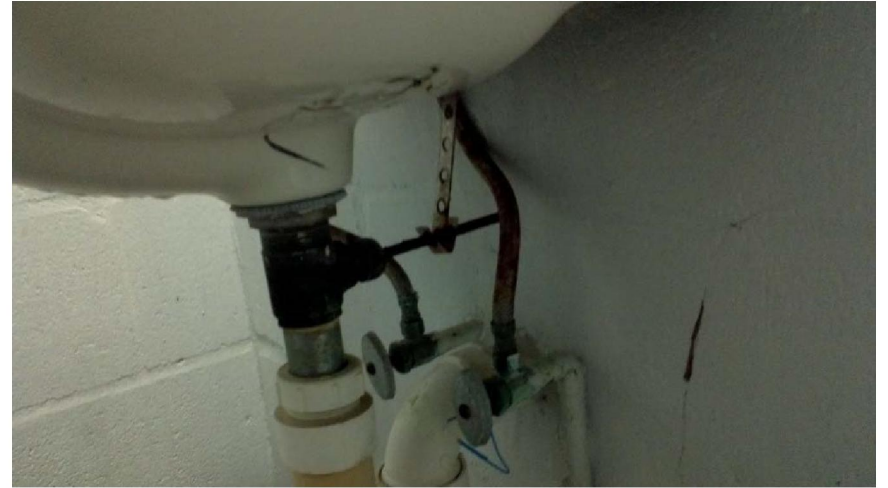
ADA violation – Piping shall be protected
