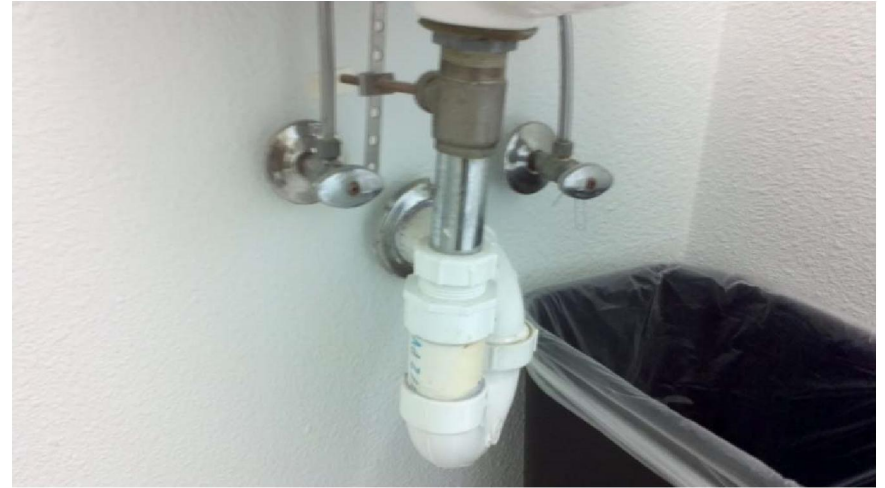
Piping is not protected per ADA
