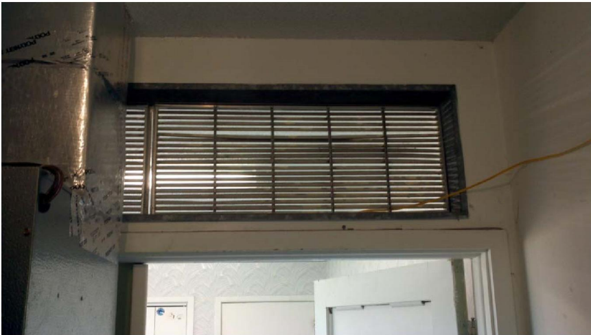
Air transfer grill to office should be ducted
