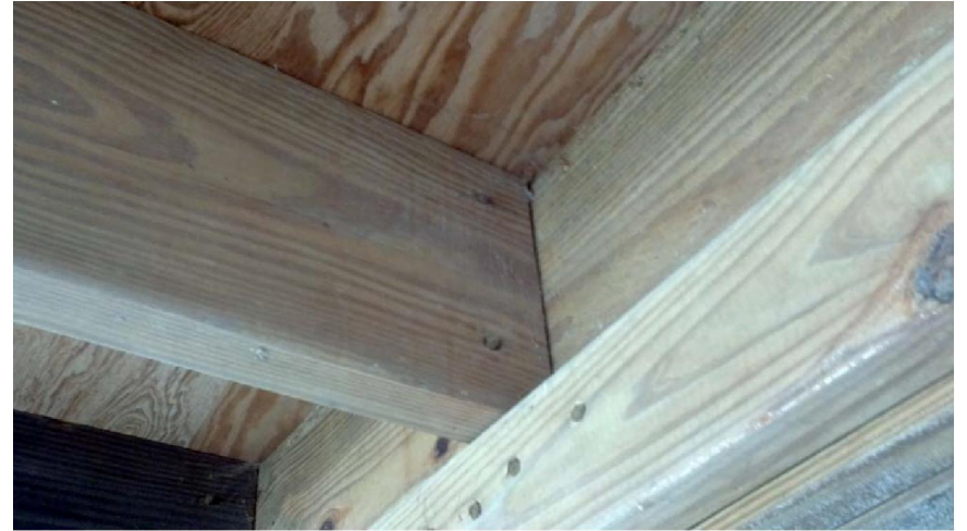
Requires proper hurricane straps and tie down
