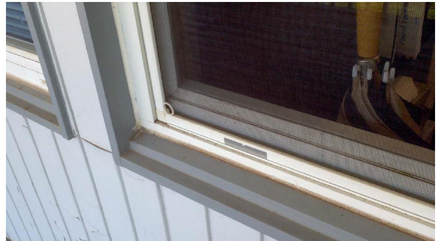
Existing glazing does not meet hurricane impact rating requirements.
