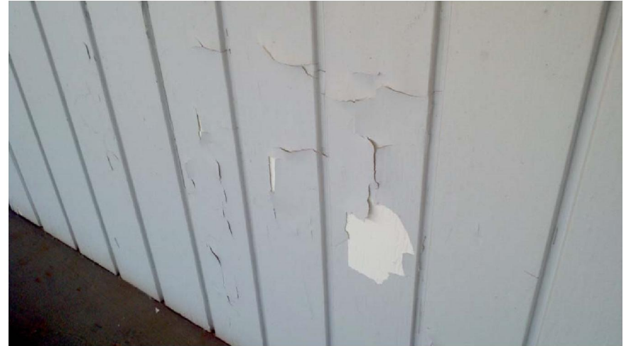
Paint delamination
