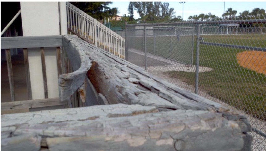
ADA Violation Railing - heights vary, no 1-1/2" continuous railing is provided. The ramp also displays a overall level of disrepair reducing functionality.
