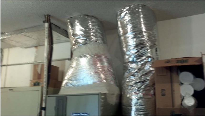
Flexible duct lengths exceed FBC requirements
