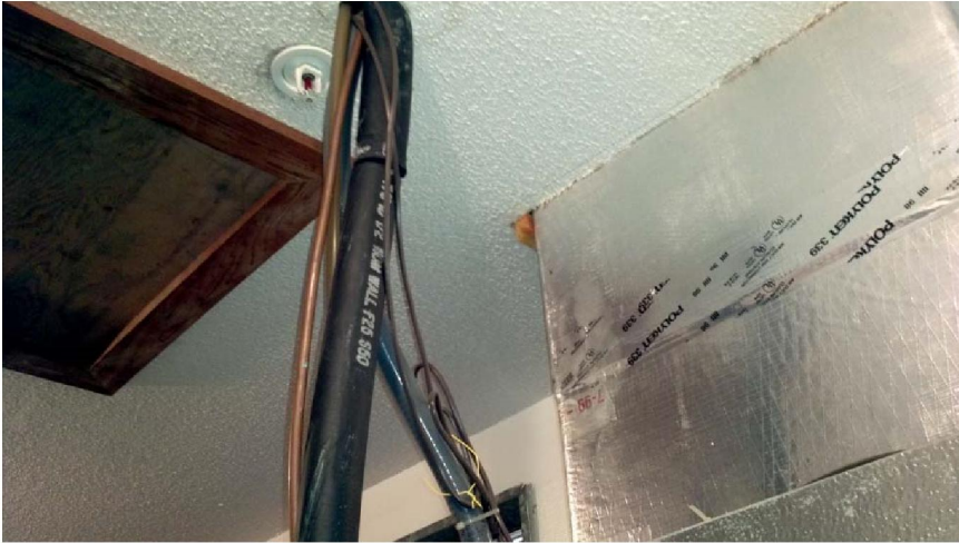
Openings not sealed between ceiling and attic
