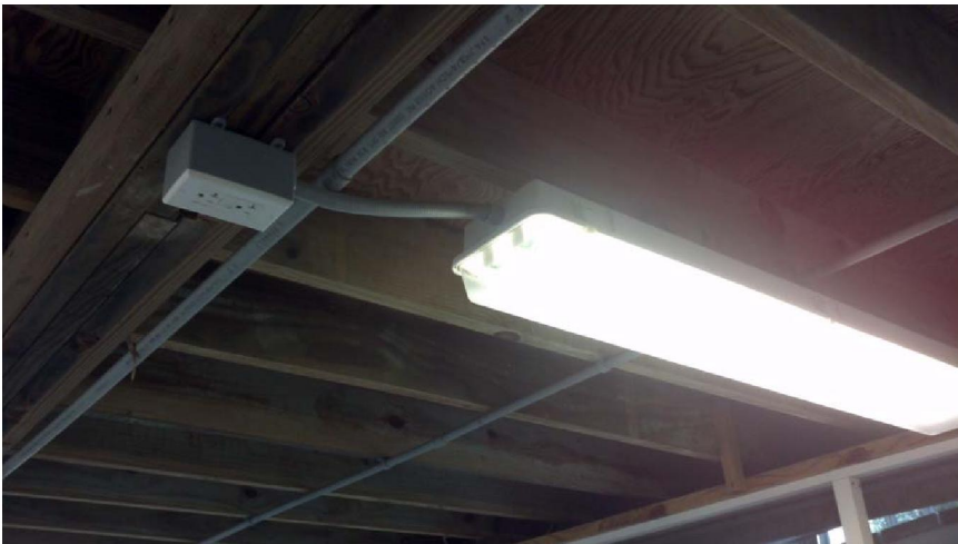
2x8 framing utilized for floor joist. 2x10min is recommended
