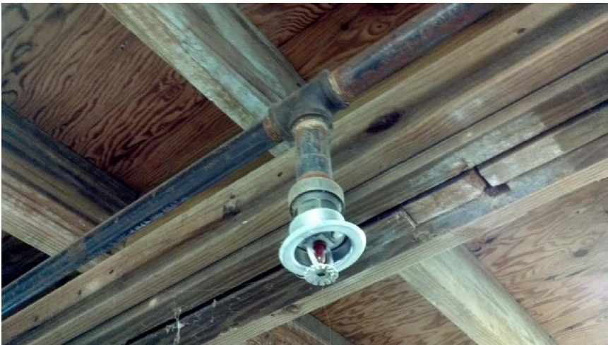
Building is sprinkled. WJA does not recommend exposed pipe in salt water locations
