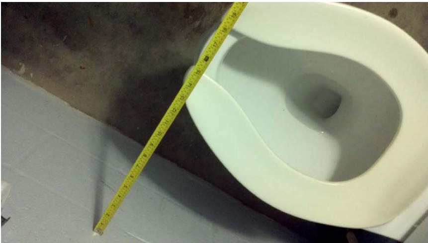
The toilet is not the correct distance from the wall per ADA
