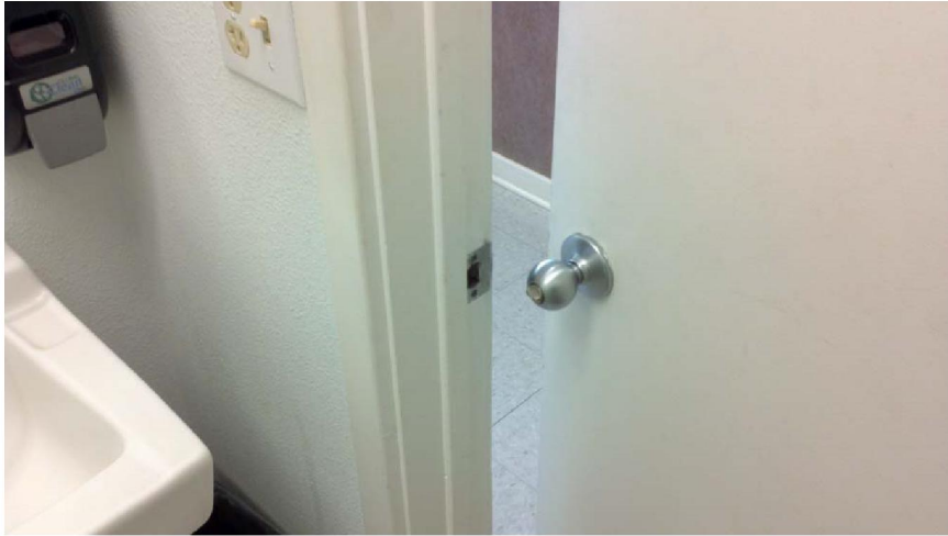
Door handle should be a lever per ADA. Push side of the door should have 12" clear
