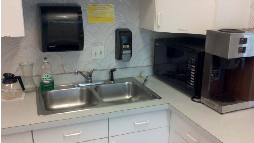
Triple bowl sink is required Separate hand sink is required
