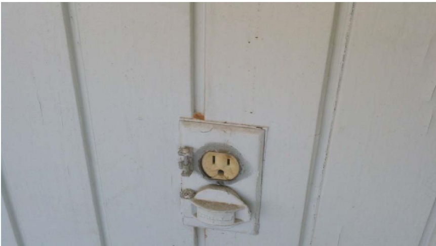
Exterior electrical fixtures do not appear to be ground fault protected. Potential liability
