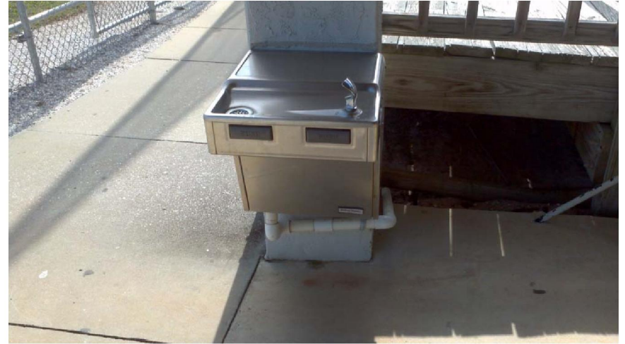
Plumbing is below flood plain without visible back flow preventer
