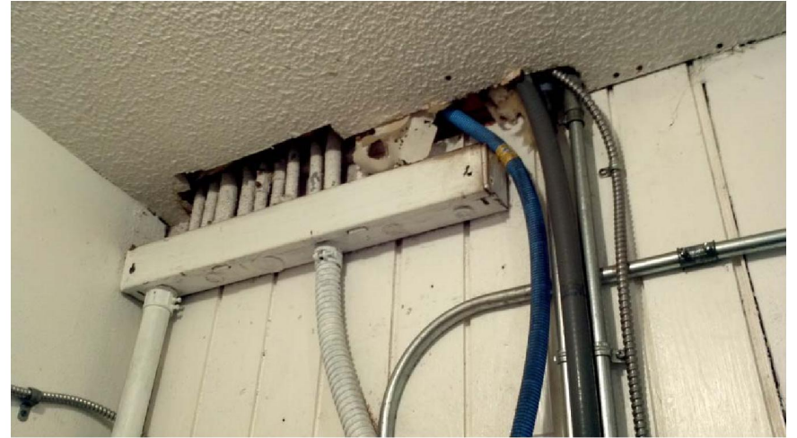
Openings not sealed between ceiling and attic
