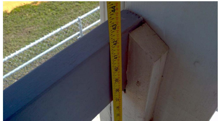
Guard rail height varies from 41-43 inches. 42" guardrail is required per FBC
