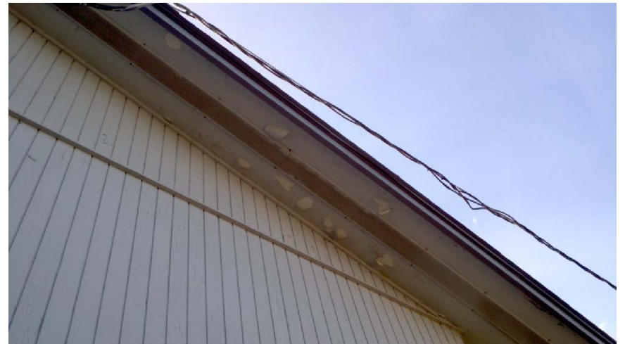
Exterior paint is peeling exposing wood siding, fascia, and sheathing
