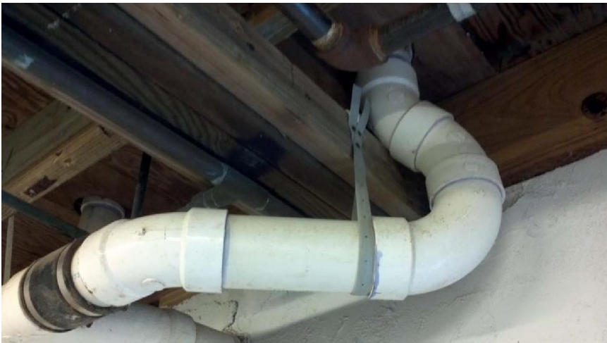
Extensive use of rubber couplings
