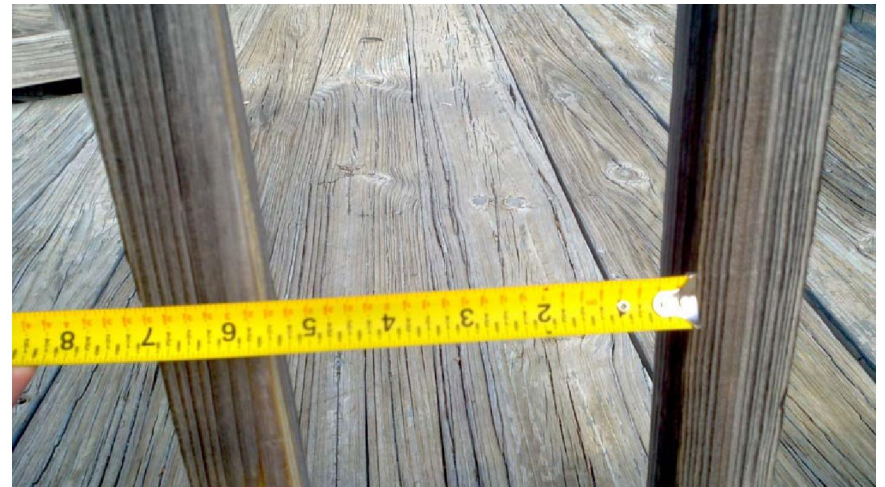
Railing should not allow a sphere greater than 4" to pass between railings. This is a liability for youth patrons.
