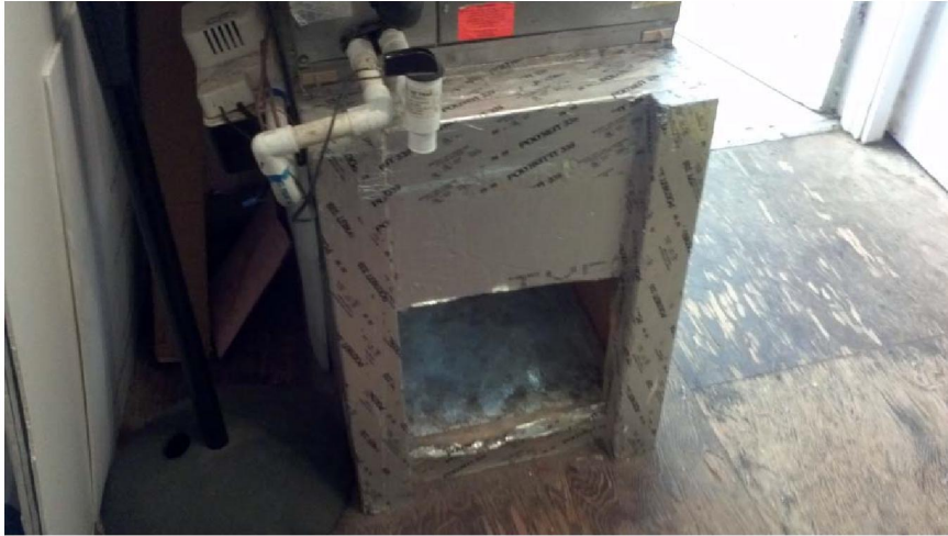
The building does not have code required ducted return air and does not meet the current outside air requirements
