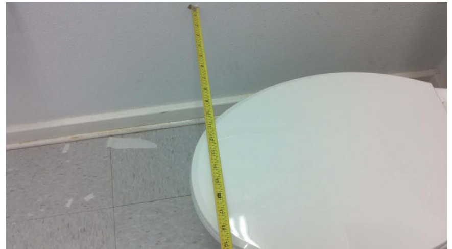
Toilet dimension does not meet min ADA dimension requirements
