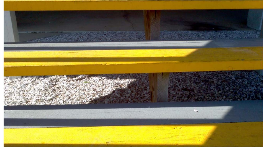
FBC Code Violation – Open tread stairs are not allowed in commercial construction.
