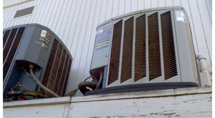
Condensers appear to be functional and have usable life available.
