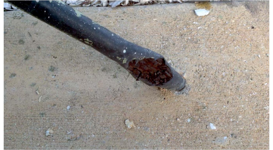
Lateral bracing is rusting through at multiple locations
