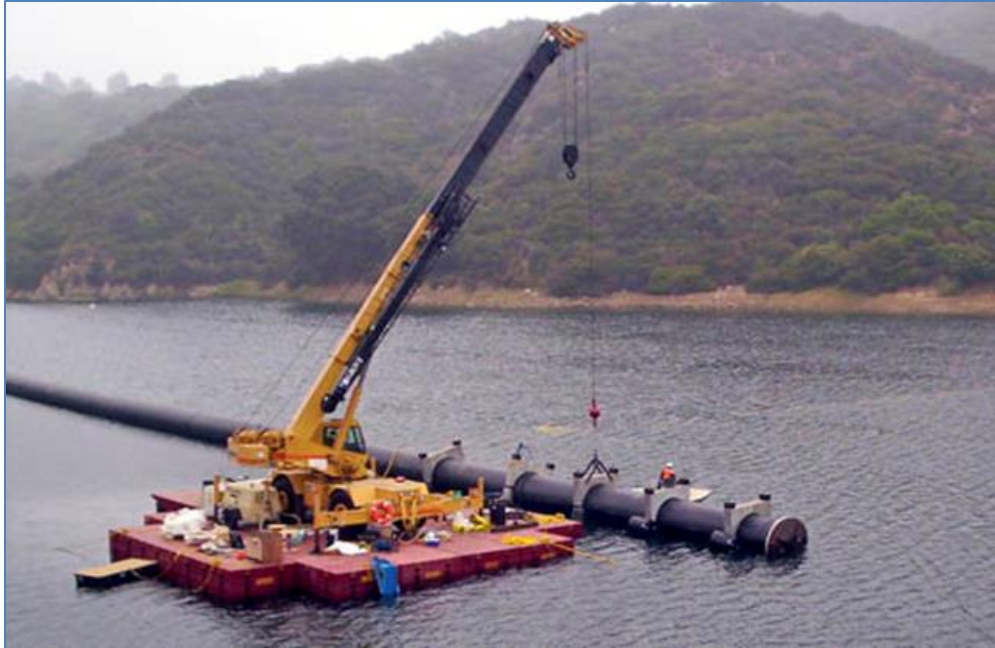
Figure 3-12 Barge Mounted Crane
