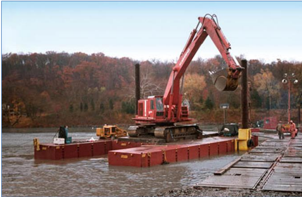
Figure 3-11 Sectional Barge with Excavator
