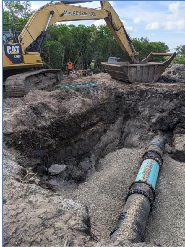
Figure 3-17 Photograph of Existing Force Main Repair
